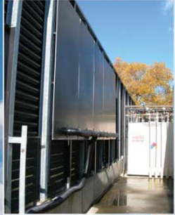
As part of the campus-wide plan to reduce engine heater electricity use, solar air Heater Boards™ were installed along fences to provide solar heated air to generator enclosures (above).
