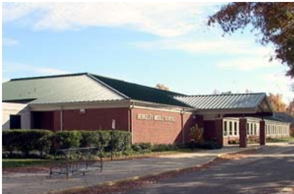
Image: Berkeley Middle School Metal Re-roof Over Flat Roof
